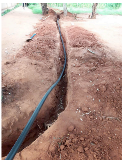
Figure 4 Laying 1Km of pipe
