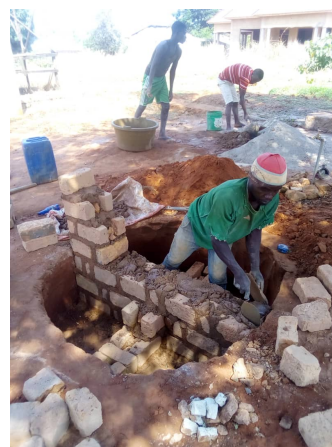
Figure 1 Building of the support tower in preparation for water tank
