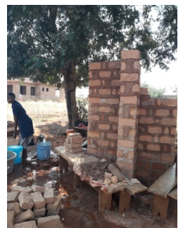
Figure 1 Building of the support tower in preparation for water tank
